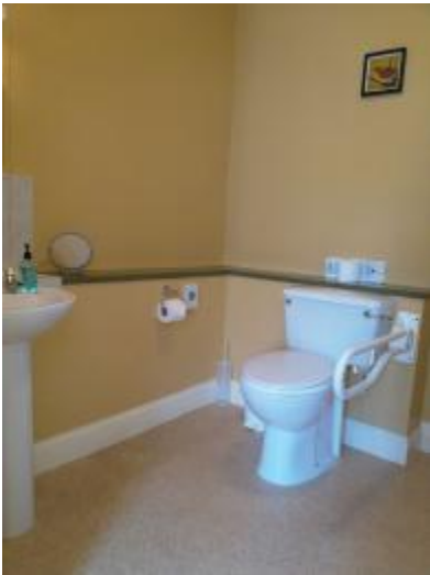
Ground floor bathroom toilet with assistance rail lowered
