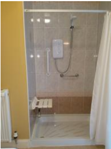
Ground floor bathroom shower with flap seat lowered and showing two grab rails
